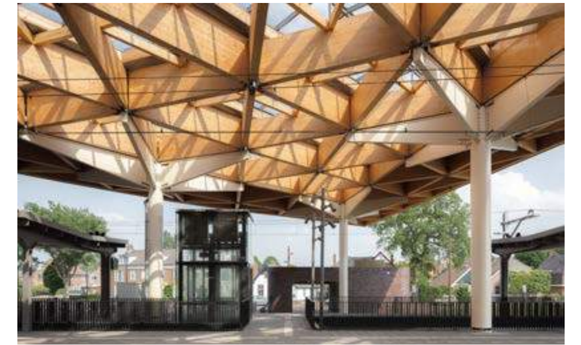
Station Assen Assen
